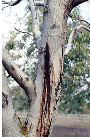
Figure 2. Symptoms of systemic infection exhibiting reddish brown exudate from cracks in trunk and limbs. (Courtesy B. Teviotdale)
